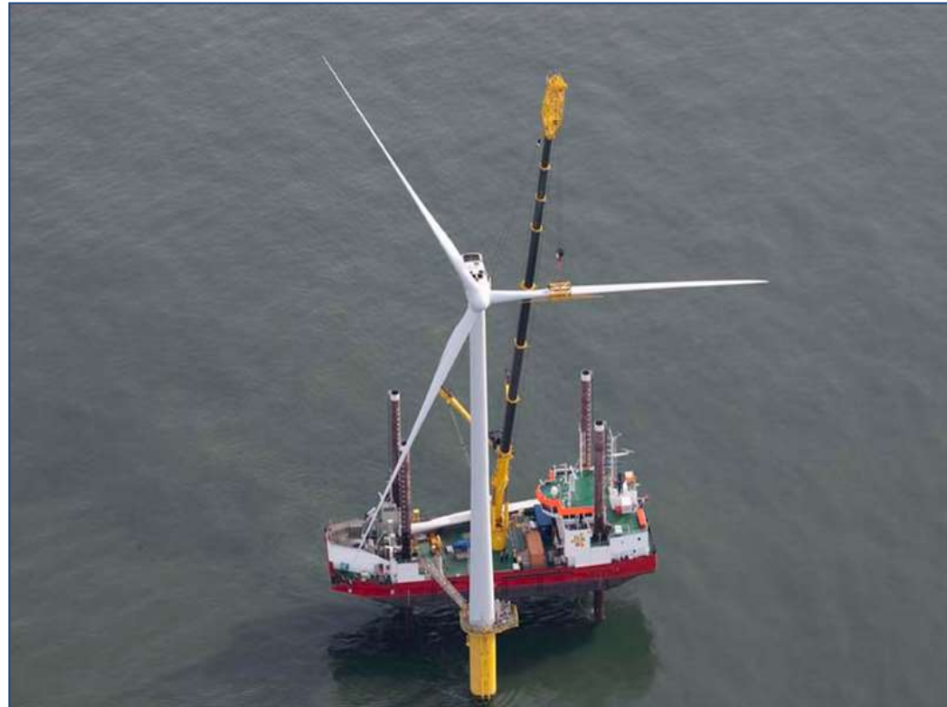
Offshore installation of blade
